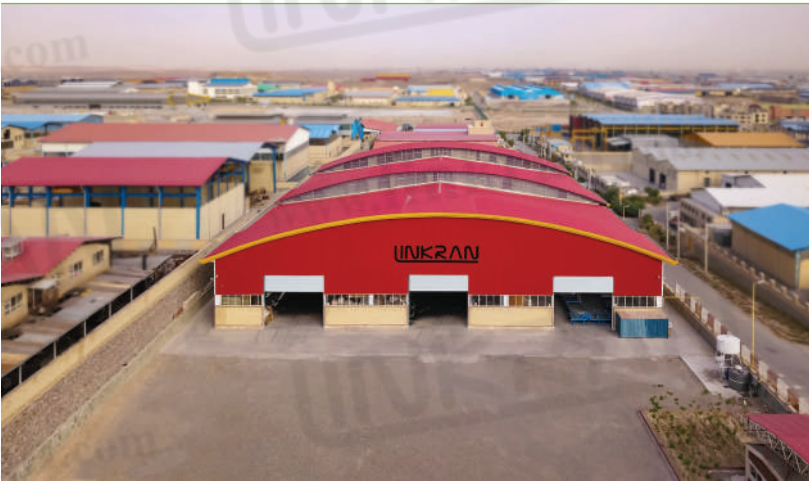
LINKRAN Site (Shams Abad Industrial Zone)
